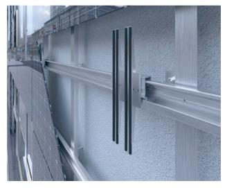
Solar Facade Systems can be installed on office and residental buildings, as well as on existing logistic centers and hubs.
